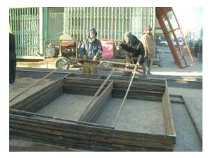
The first step of metal guy was to stand up the wall it takes almost 8 days. After that the next step was to covering of the roof. When he did complete the wall than he started the final step which was roof of the room.
